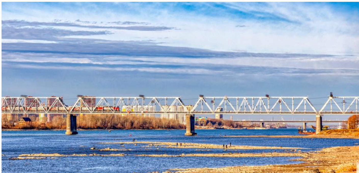
Railroad bridge over the Ob' River (Source: Dmitry Karyshev on Flickr.com)
