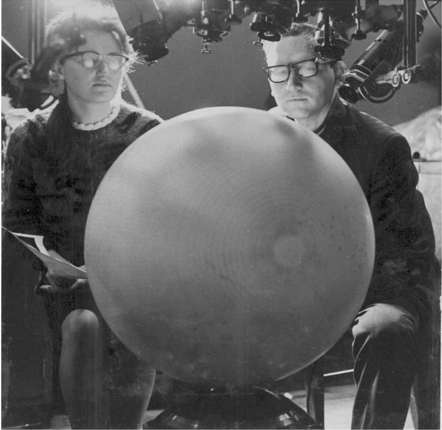
**Fig. 2.10** Zh. F. Rodionova and V. I. Chikmachev in the Department of Lunar and Planetary Physics (GAISH) working with the unified multiplex apparatus, equipped with a precision spherical screen for tying the coordinate systems of spacecraft images
