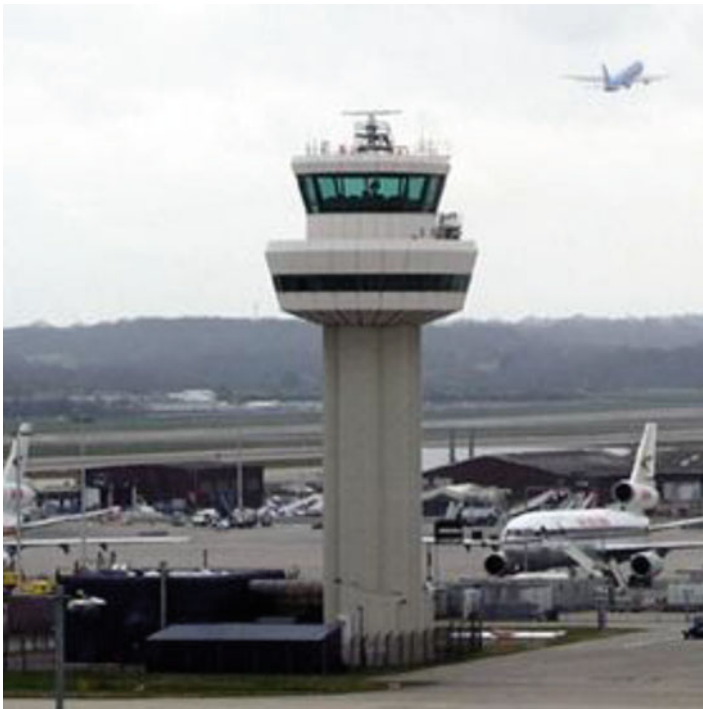
Fig. 2.12 Typical air control tower ( www.wikipedia.com )
